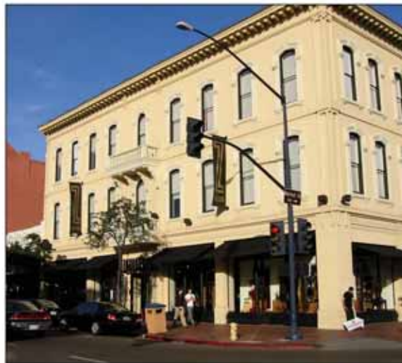
Corner Shopfronts in Commercial Block building
